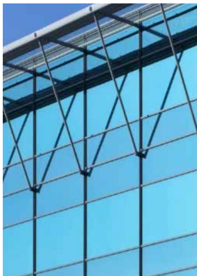
Figur 28: Semitransparenta solceller i glasfasad (SolTech).
